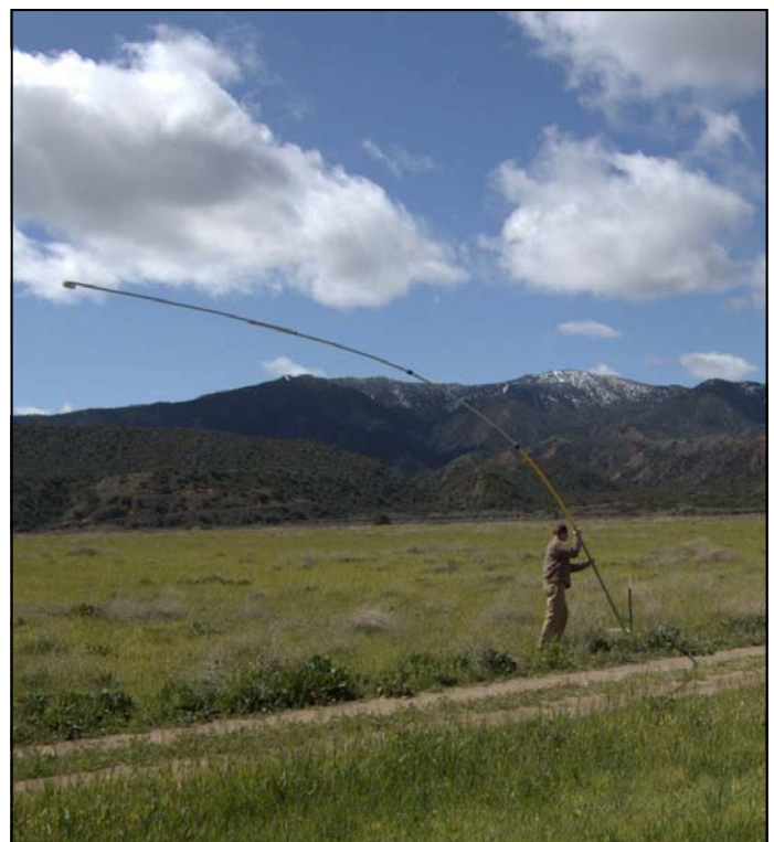
Figure 2. The author installing one of the 35 ft. meteorological towers at the Cuyama site.
