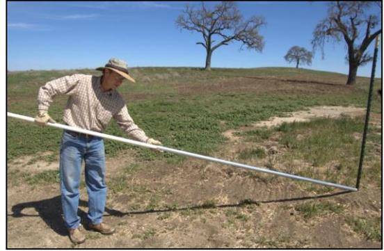
Insert the bottom end of the "Mr. Longarm" into the line post; it should insert 2 ft. inside the post, and the band of "Gorilla" tape should be fully inserted inside the line post with a close fit. If the fit is too loose, add more "Gorilla" tape; if too tight, remove some of the tape.
