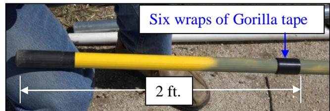
Using the “Gorilla” tape, make six complete wraps around the pole, with the upper edge of the tape aligned with the pencil mark. The outside diameter of the finished taped section should be slightly smaller than the inside diameter of the steel line post, into which it will be inserted later.
